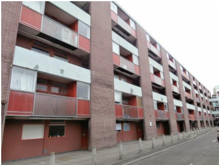
Basterfield House northern elevation
